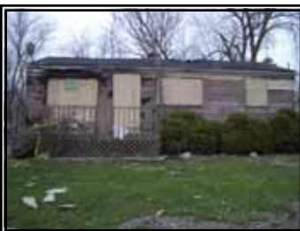
City of Pontiac Spot Slum and Blight Demolition Program—85 Gillespie, 81 Lake and 877 Melrose demolished during the reporting year.
