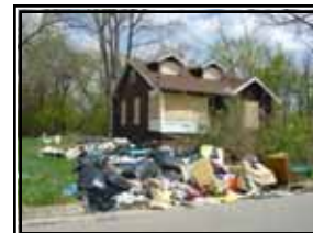
Abandoned home at 155 Howard McNeil demolished by the City
